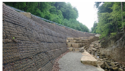
Figure 8: Stabilisation system under construction.
